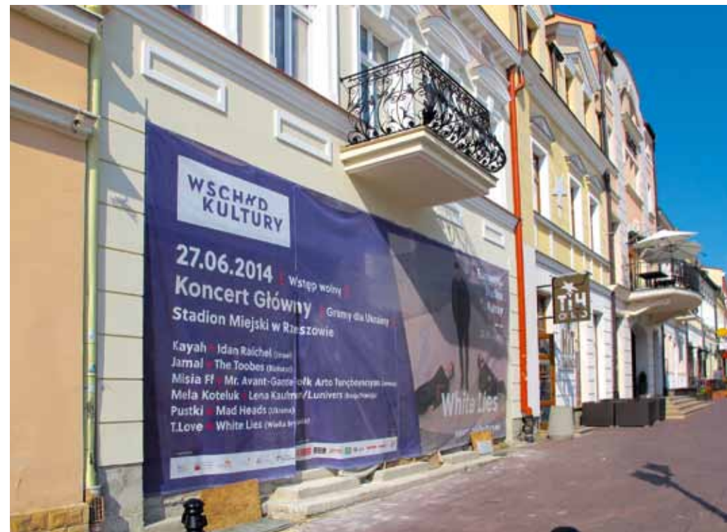
BANNER COVERING A BUILDING IN THE PROCESS OF RENOVATION
