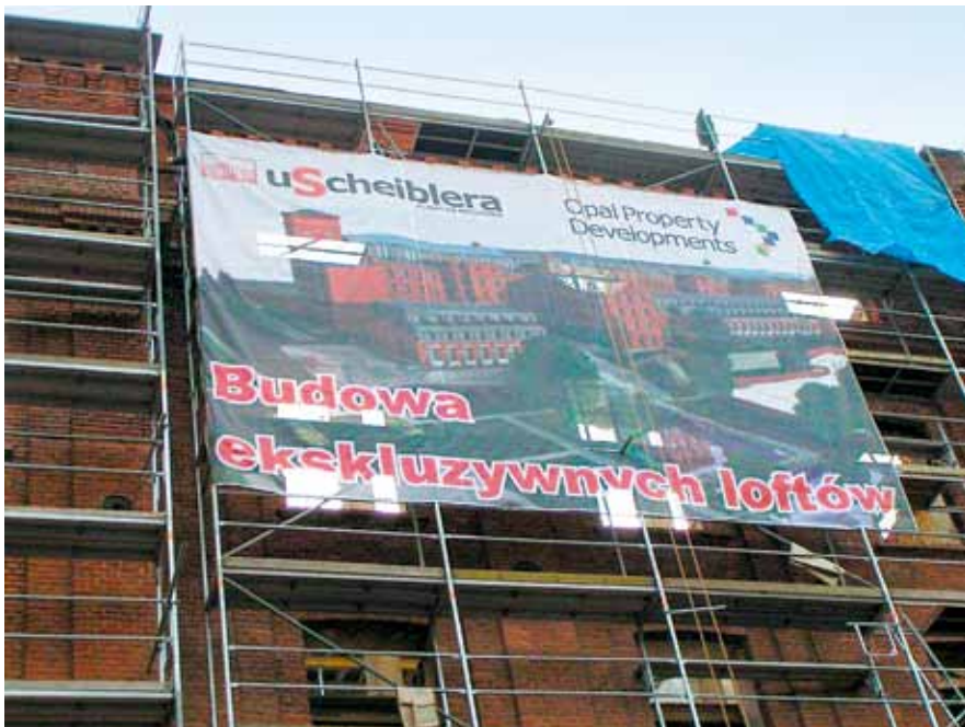
TEMPORARY ADVERTISING BANNER ATTACHED TO SCAFFOLDING
