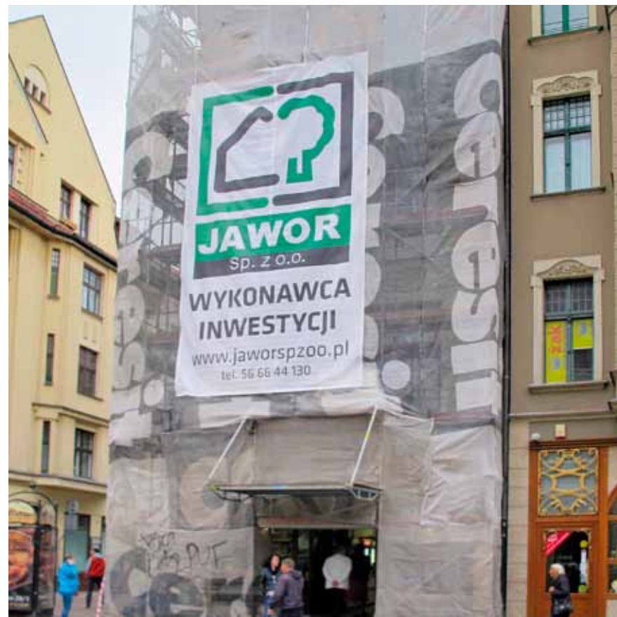
TEMPORARY ADVERTISING BANNER ATTACHED TO SCAFFOLDING
